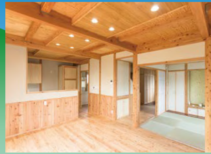
To improve the usage rate of Hokkaido-grown timber, we have recommended the use of Japanese larches for structural and interior materials, and verified its quality with demonstration tests using an actual house.
