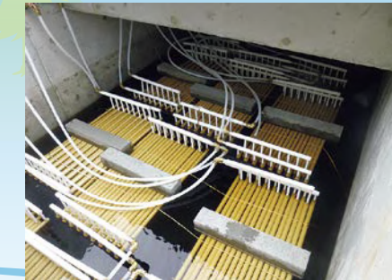
In collaboration with a Hokkaido company, we have developed an easily cleaned plastic heat exchanger that can recover heat from strongly acidic hot spring water or dirty hot waste water with many suspended solids. It is applied to a preheating hot-water supply system.
