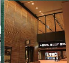
Fire proofing ash
