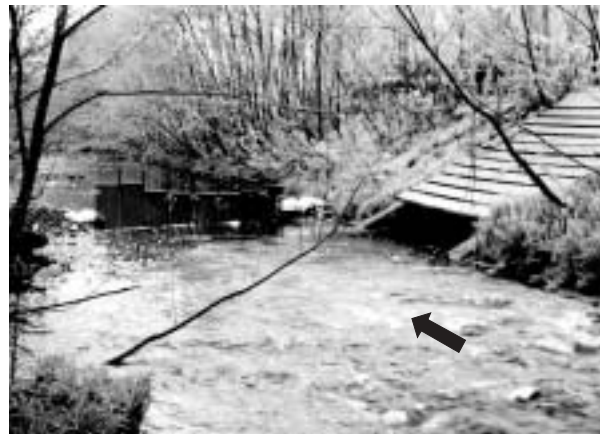
Fig. 22 A partial fence installed above the Soya Research Branch of the Hokkaido Fish Hatchery. The arrow indicates flow direction.
