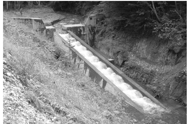
Fig.4 The new fish way of S42 groundsel constructed in 2013.
