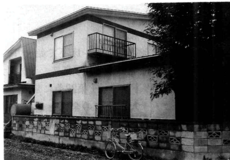
写真5 調査家屋 [ケース 2] 外観 Photo.5. The outside appearance of the house surveyed , case 2 .
