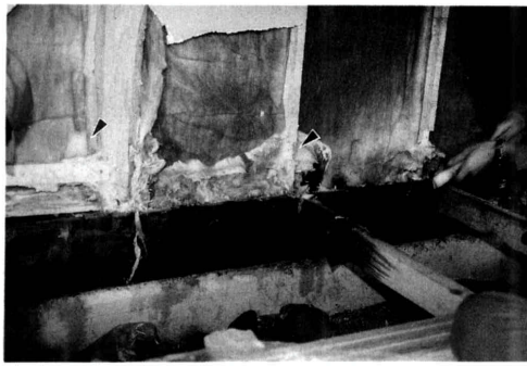
写真 13 壁内結露を生じた部分での菌糸生長 (▶) Photo . 13 . Hyphal growth (▶) inside the wall in which the condensation moisture occurred .
