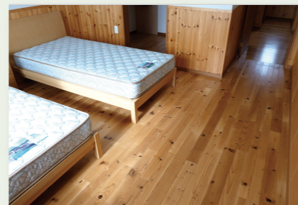
Compressed Fir wood Aiming for using fir as interior material, compressed wooden flooring having the same level of functionality with hardwood is being developed. Patent No. 5629863
