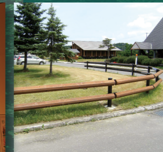
Crash barrier made of Hokkaido wood
