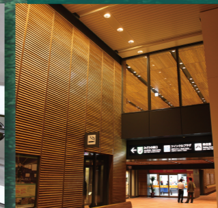
Fire proofing ash
