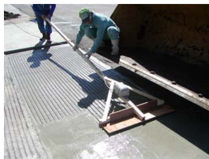
(牛舎通路の溝の施行)
