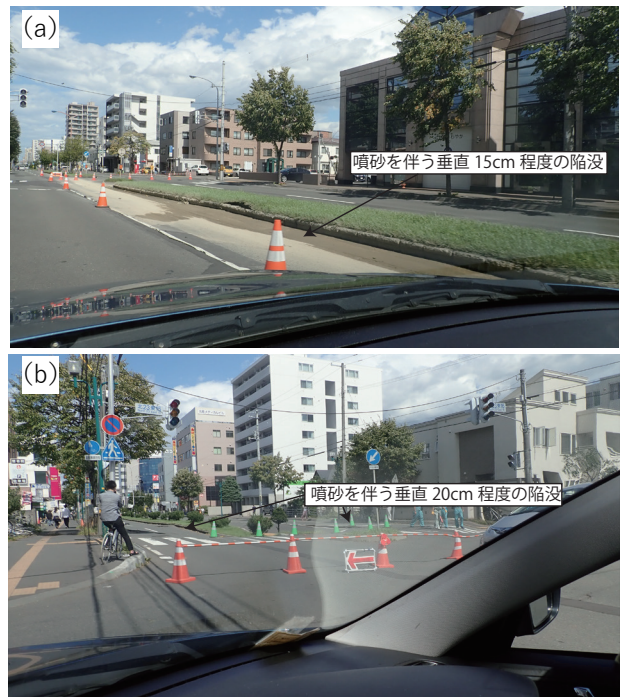
図6 東区北13条～北24条にかけての地盤変状状況 Fig. 6 Destruction situation of surface rupture between kita-13 jo and kita-24 jo, higashi-ku, Sapporo city.
