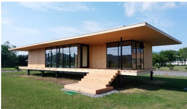
写真2 Hokkaido CLT Pavilion (CLT実験棟)
